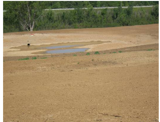
Figure 4. Sedimentation pond – wetlands & adjacent area ready for seeding.
