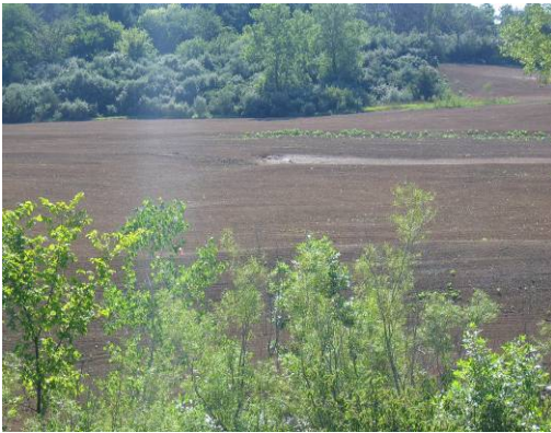
Figure 3. Topsoiled & ready for seeding.
